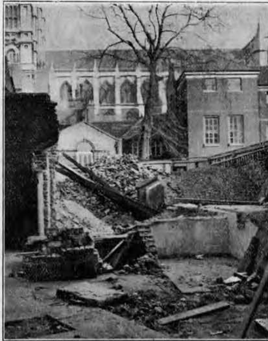
The Demolition of the Fives Courts in Yard; part of the plans for preparing No. 17, Dean's Yard for use as a School Building.
